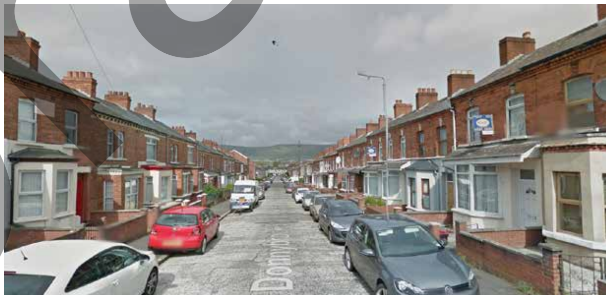
Figure 12. SuDS integrated into a typical Victorian terrace example - Street view, Belfast
